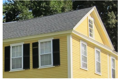
Window casings, corner board, cornice
