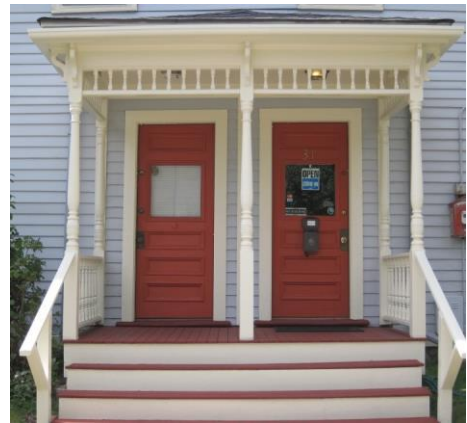
Paneled doors with square lights
