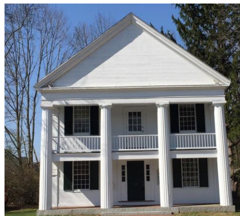
Wood flushboard siding in gable peak
