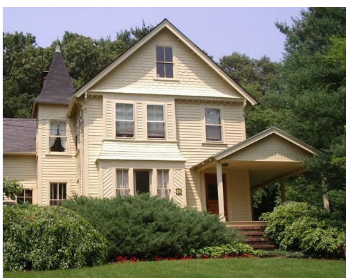
Patterned shingles and clapboards
