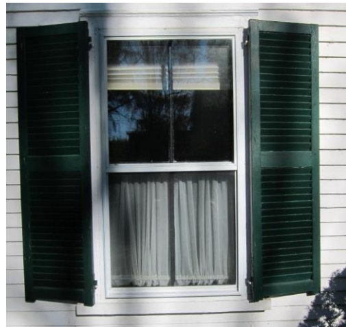
2/2 double hung sash with exterior storm
