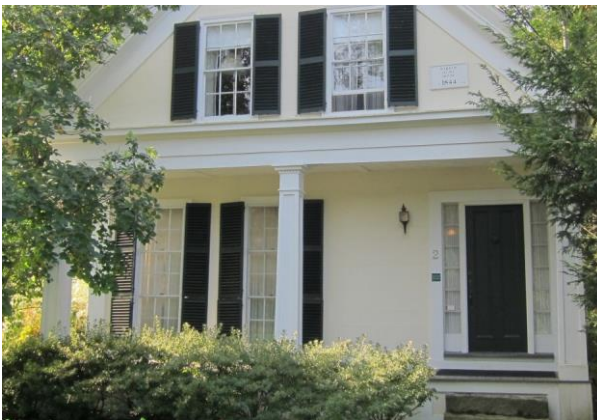
Full length wood louvered shutters flank windows
