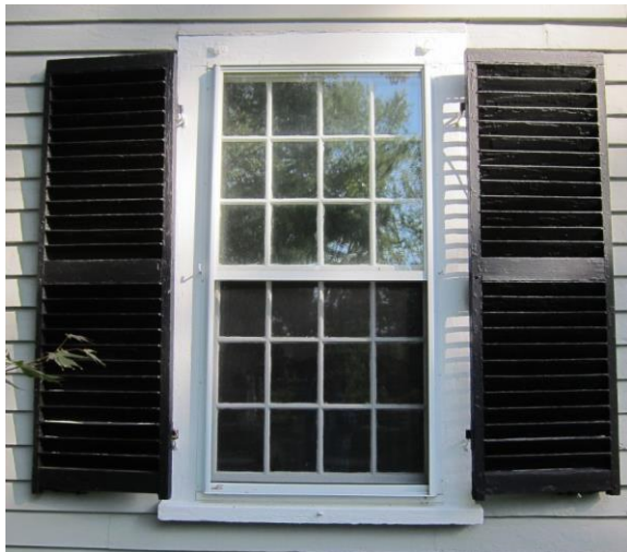
12/12 double hung sash with exterior storm
