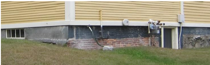
Mixture of brick, stone and granite foundation
