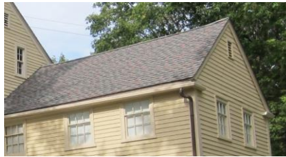
Asphalt shingle roof
