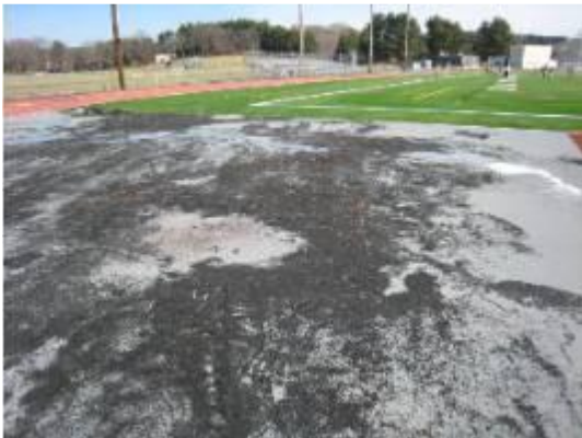
Figure 15 - Photo: Degraded Crumb Rubber
